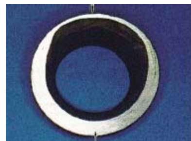
Internal wall thinning in a pipe subject to FAC.
